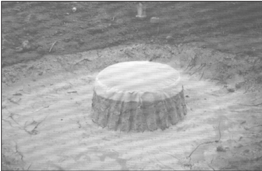
Figure 6-28.7 Equivalent Inlet Sediment Trap
