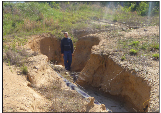
Figure 1.1 - Advanced gully erosion on an abandoned construction site.
