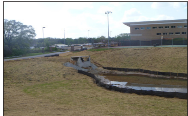
Figure 2.11 - This temporary sediment basin effectively trapped sediment from upstream erosion.
