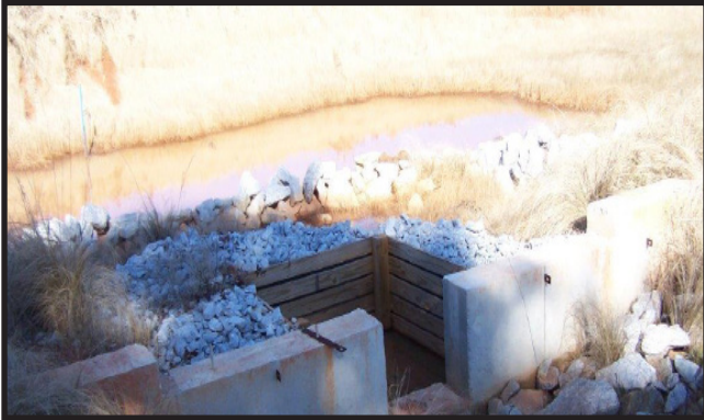
Example of Slotted Board Dam
