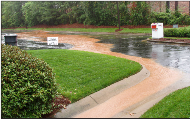
Figure 2.13 - Offsite impact from a neighboring construction site.
