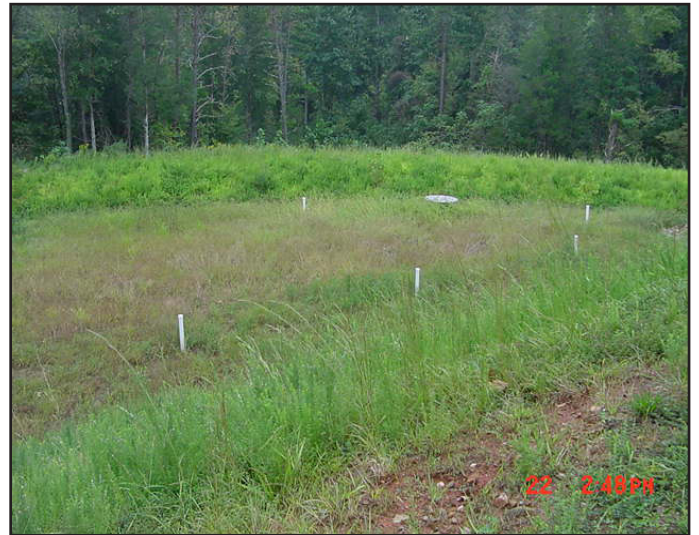
Conversion of a sediment basin to a bioretention area. The original riser acts as the overflow structure for the bioretention practice.
