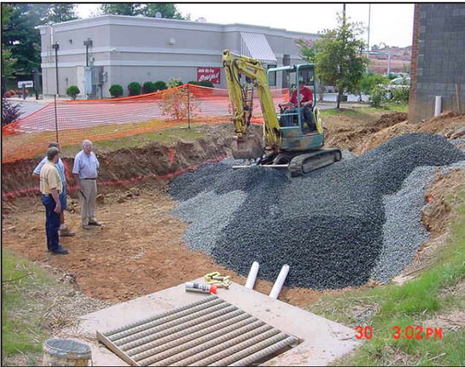
Conversion of a small-scale sediment trap to bioretention. The photos shows adding an underdrain system.
