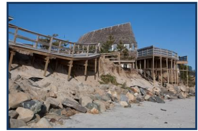
Severe beach erosion and damage resulting from a nor'easter.
