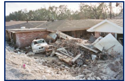
Canal levee breaches as a result of Hurricane Katrina in New Orleans in 2005. Note damages can be more extensive due to high velocity flood flows than if the levee was not there.
