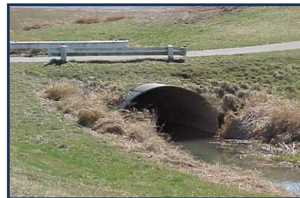
Before Mitigation and After Mitigation
