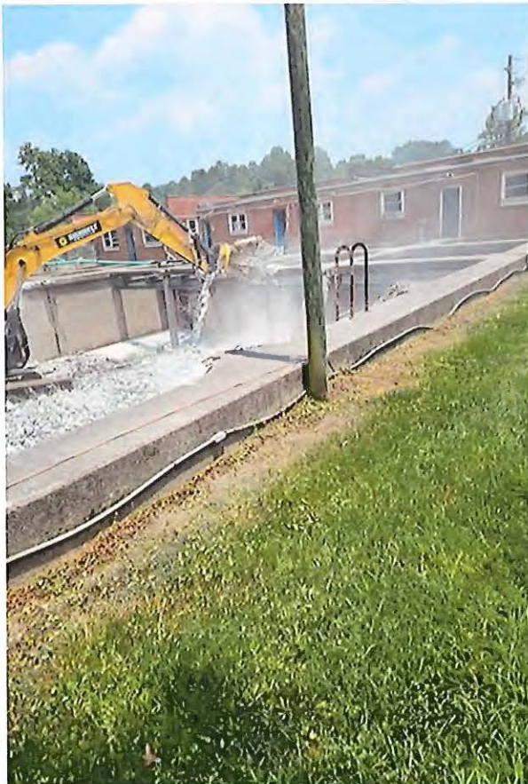
Filter Basin at Old Water Plant
